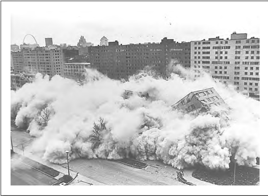
Figure 5.1 The Demolition of the Pruitt-Igoe Housing Project in St. Louis
