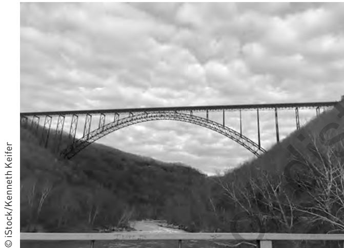
FIGURE 9.1 ■ New River Valley Gorge Bridge
